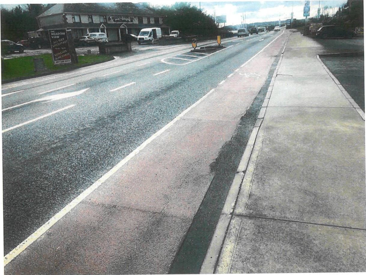
PHOTOGRAPH NO. 2: SIGHTLINE TO THE RIGHT ALONG R212 DUBLIN ROAD FOR EXITING DRIVERS
