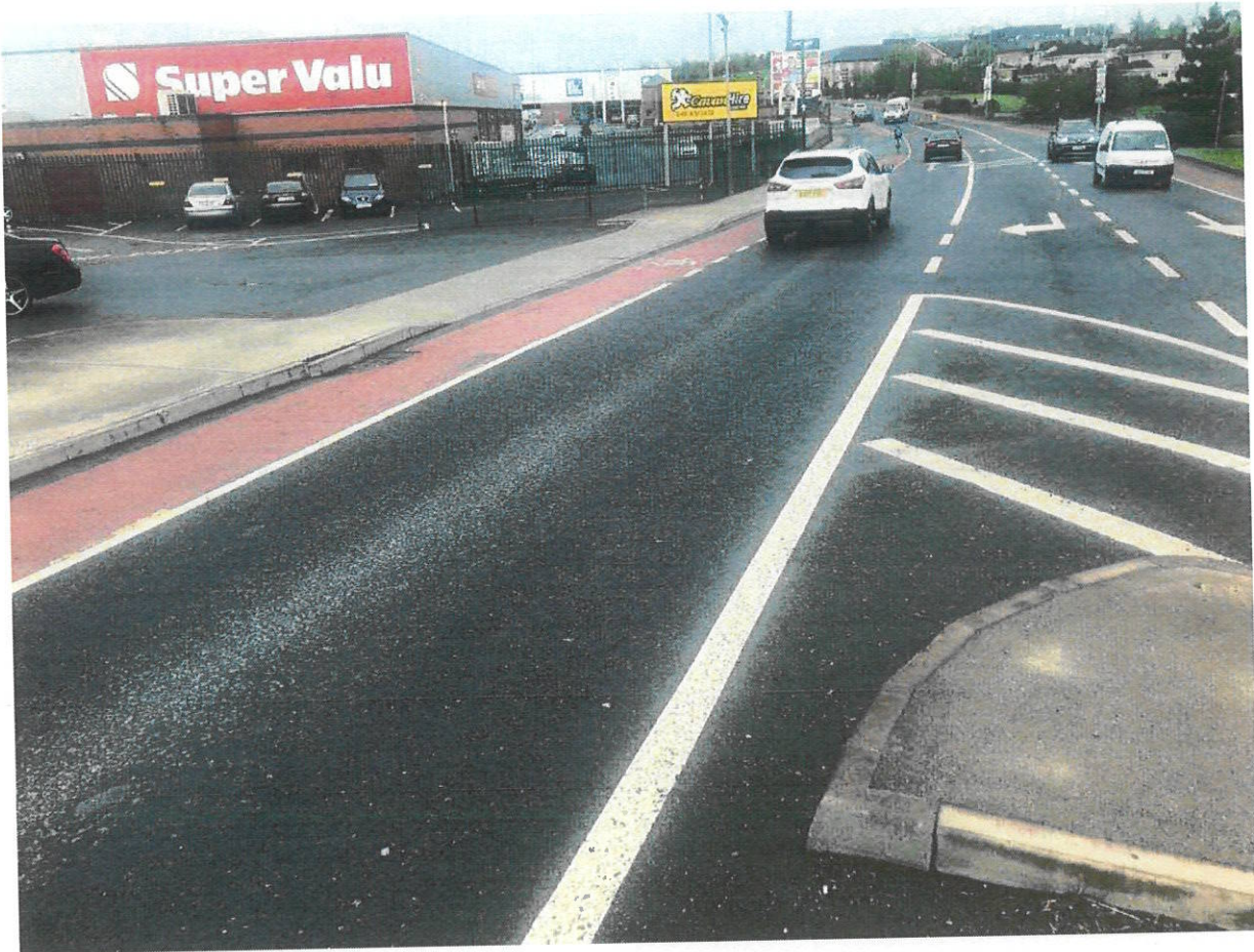
PHOTOGRAPH NO. 1: SIGHTLINE TO THE LEFT ALONG R212 DUBLIN ROAD FOR EXITING DRIVERS AND EXISTENCE OF GHOST-ISLAND LANE FOR RIGHT-TURNING INBOUND TRAFFIC
